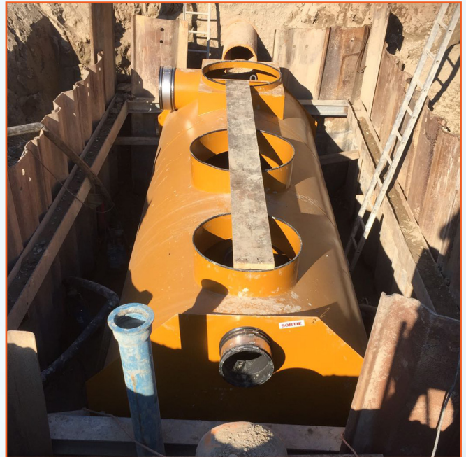
Factory Rastatt– GERMANY Treatment plan 30 l/s
